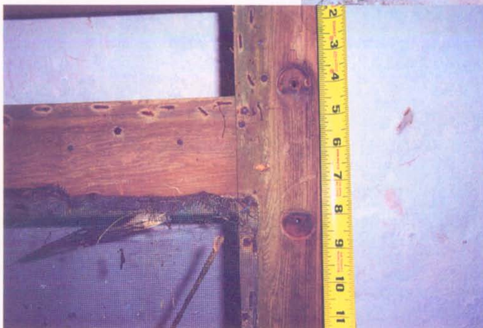
Photograph 16: DETAIL OF SCREEN DOOR SHOWING EVIDENCE OF DOOR HANDLE.
