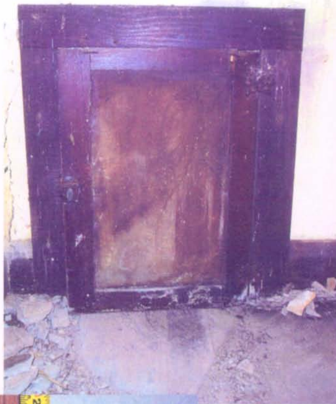
Photograph 15: DETAIL OF SECOND FLOOR ACCESS DOOR TO BATHROOM PLUMBING.
