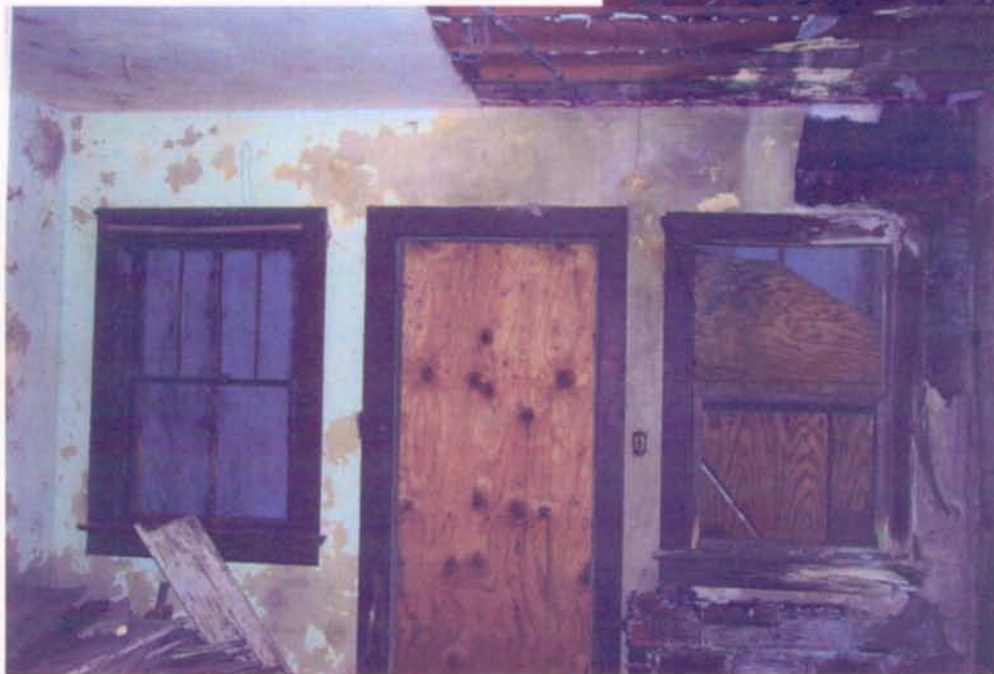
Photograph 8: INTERIOR ELEVATION OF NORTH WALL OF FIRST FLOOR LIVING ROOM.
