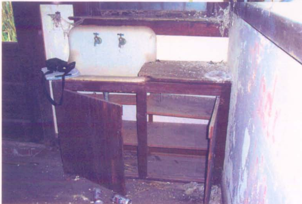
Photograph 14: DETAIL OF ORIGINAL SINK AND BASE CABINET IN WEST UNIT KITCHEN.
